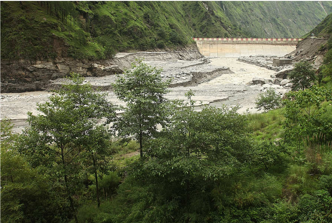
Figure 3: The Dhauliganga dam at eye-level. Note highest cut-away sand terrace on the true-left.
