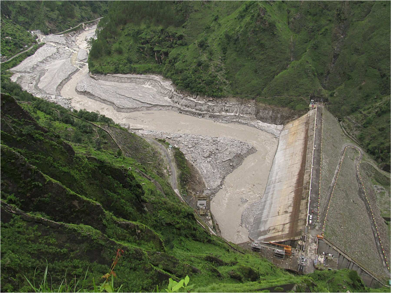
Figure 2: The Dhauliganga Hydro-power dam, after being flushed of bed-load sediment.
